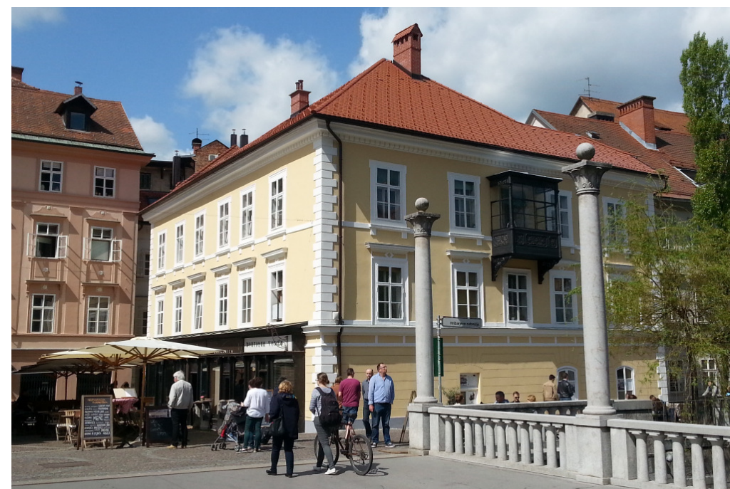
Stavba Jurčičev trg 3 pred in po obnovi; Foto: Karel Pollak The building on Jurčičev trg 3 before and after the renovation; Photo: Karel Pollak
